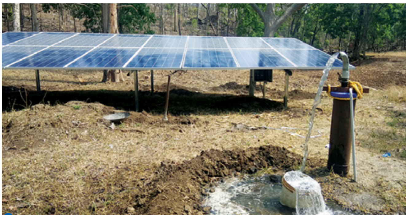
Installation of solar pumps in wildlife sanctuaries
